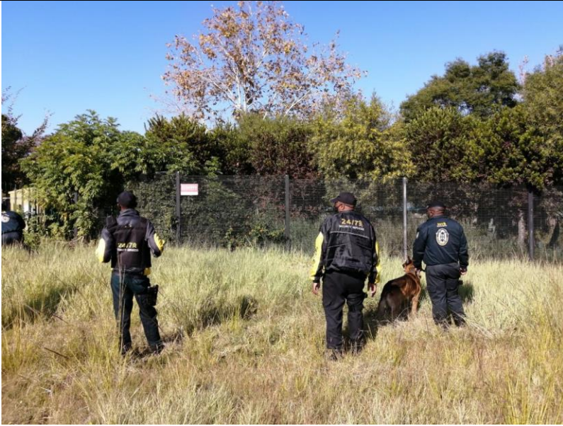
Fig 6: The perimeter compromised by overgrown foliage
