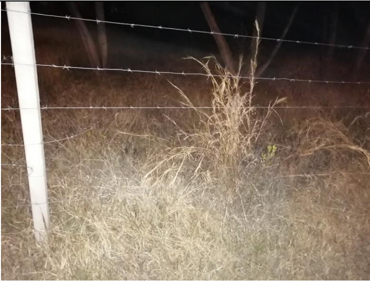
Fig 2: The Barbed wire fence is still compromised in several places.
